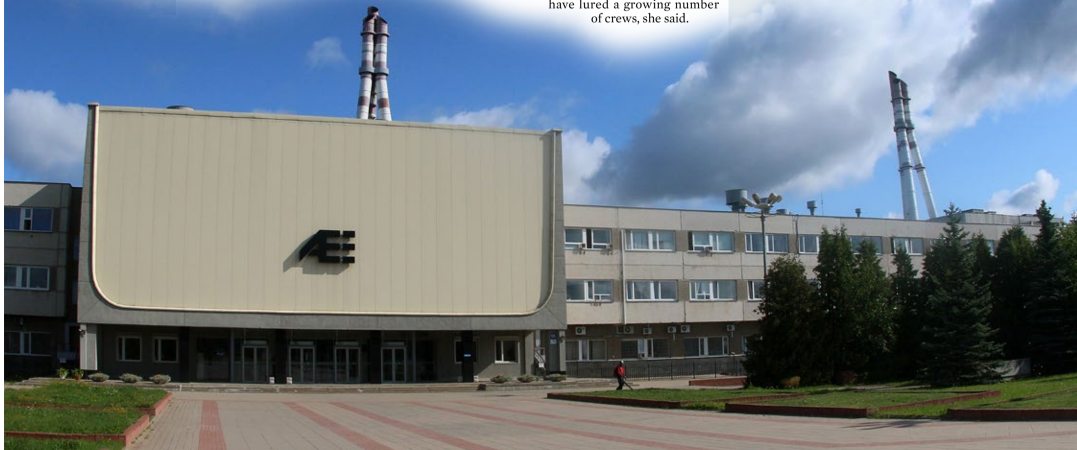
The Ignalina nuclear power plant is pictured in Visaginas, Lithuania
